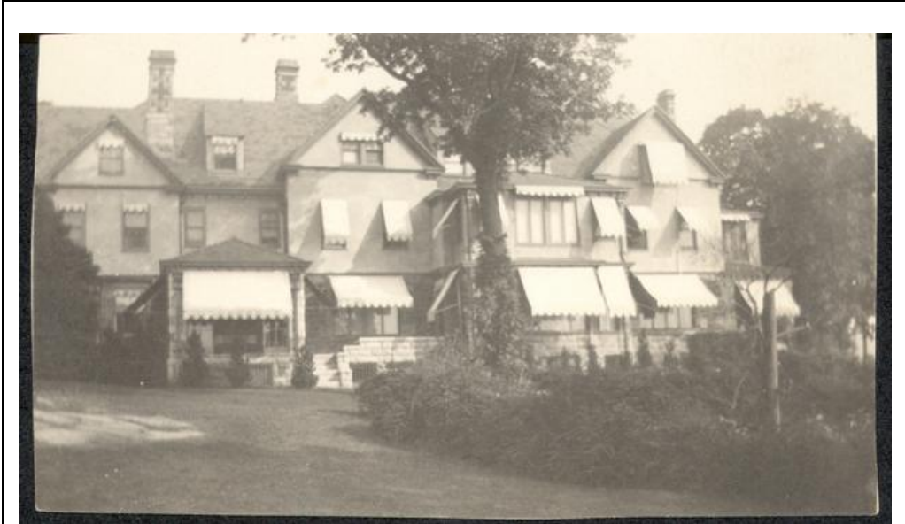
1935.11.19 Demolition of Ringling House (Gray Crag)
